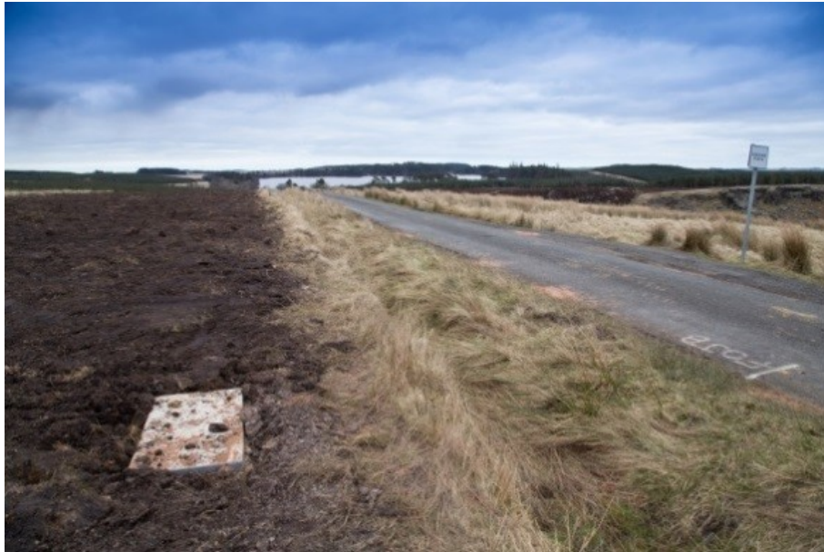
Plate 2 Example below ground link box following reinstatement (Source: Rey Wind Farm, VWPL.)
